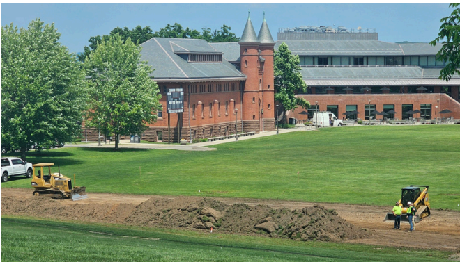
2024 installation of hot water heating pipes
