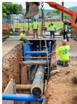
2022 installation of hot water heating pipes
