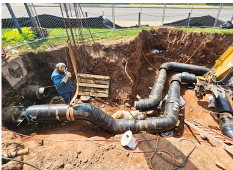
2022 installation of hot water heating pipes
